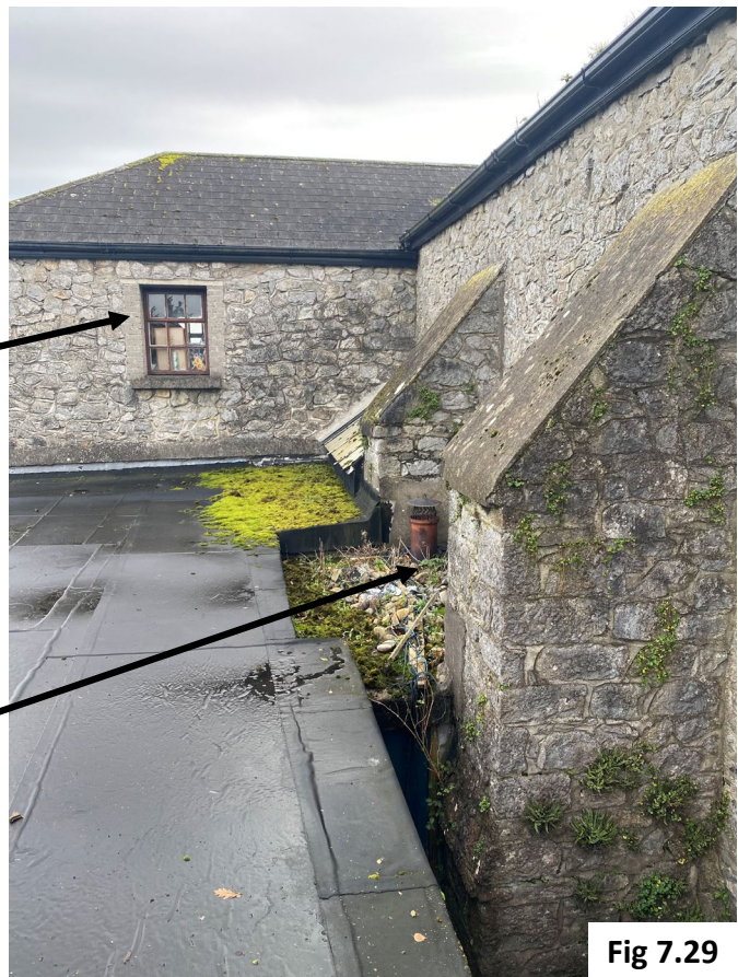
Fig. 7.29 Condition of flat roof adjoining Roof 2
